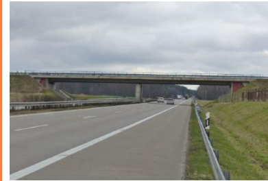
Brücke 2 Mecklenburg-Vorp. CEM I+CEM III/A Bj. 2008
